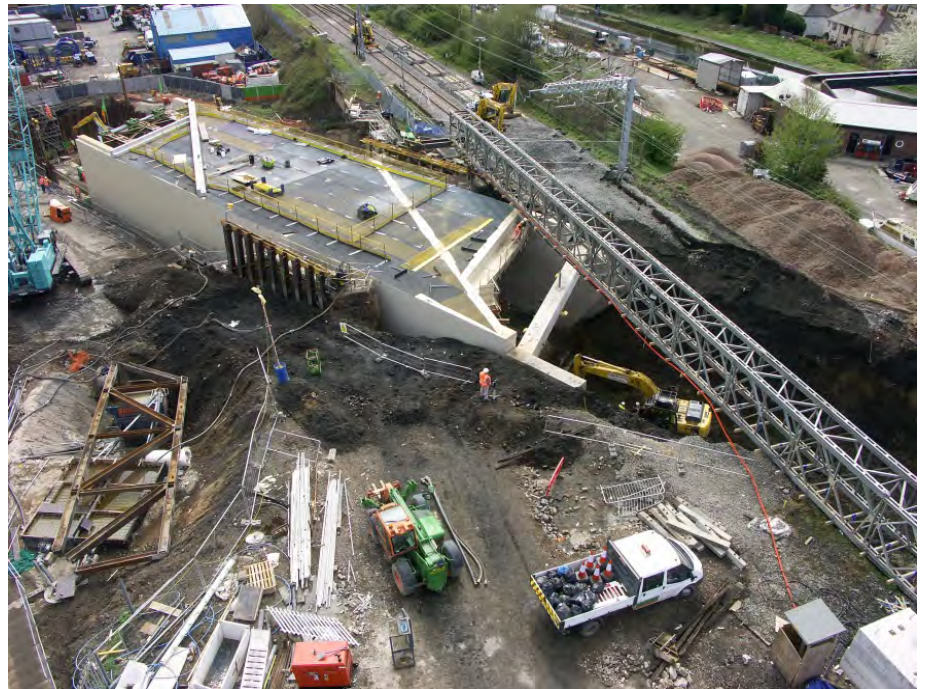
Photo 1.4: Owen Street during main possession for installation.
