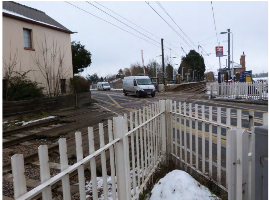
Photo 1.2: Foxton Level crossing looking north-east
