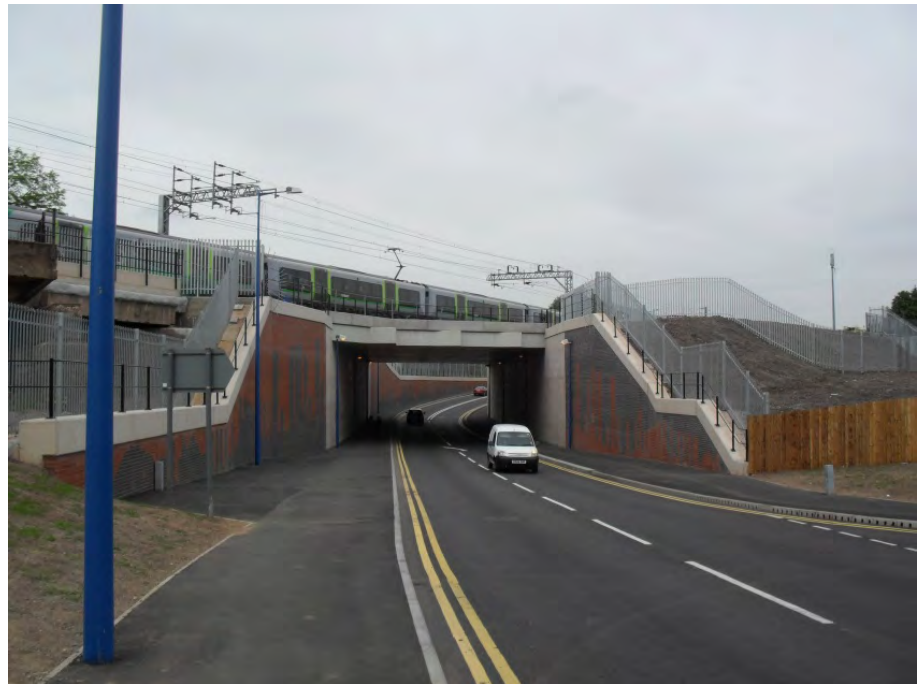
Photo 1.5 – Owen Street Underpass after completion.
